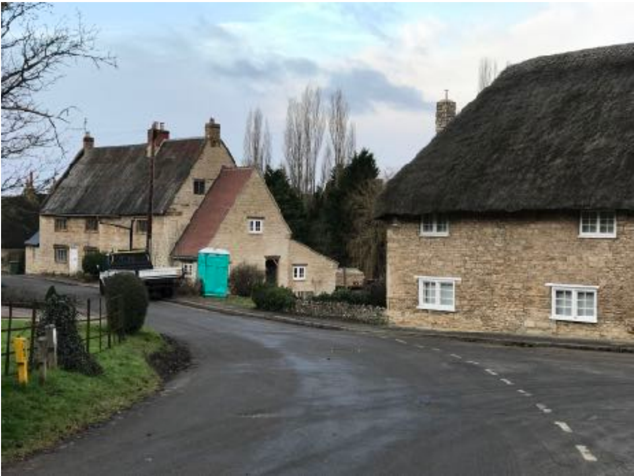
No 14 Combrook with new side and rear extension nearing completion
