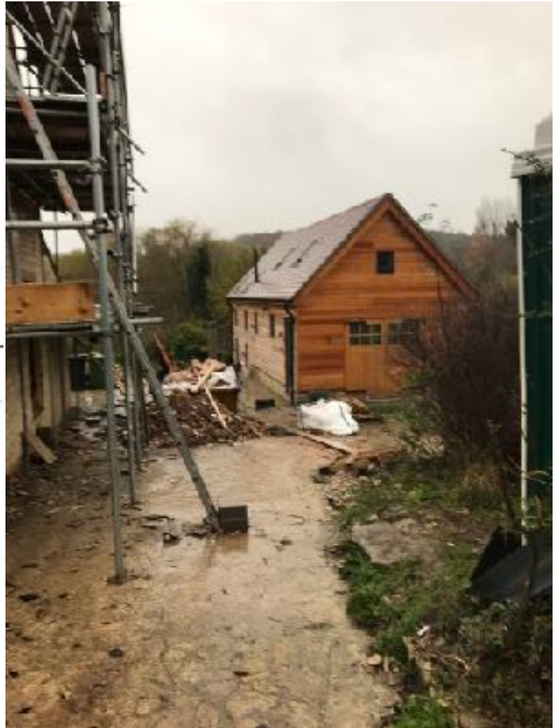
The "replacement outbuilding" as built
